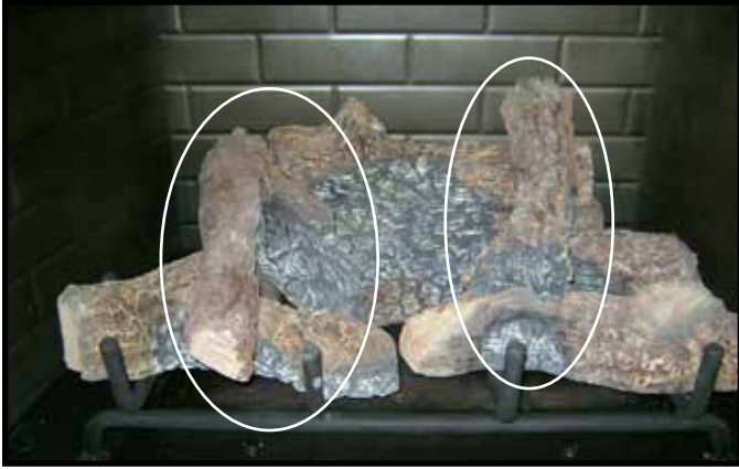
Figure 3.2 Remove Top Two Logs
