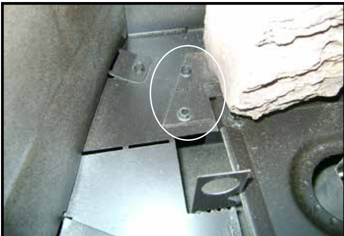
Figure 3.4 Remove Screws from Log Tabs
