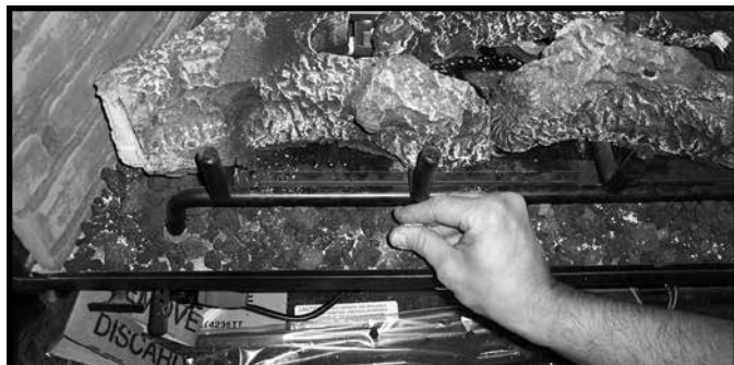
Figure 14.4 Placement of Vermiculite
